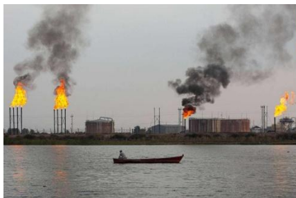
Figure 1 – The flares in the refinery
